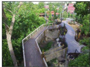
Elevated boardwalk over Emigration Creek
