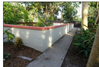
Filtration Marsh exhibit – South edge of exhibit
